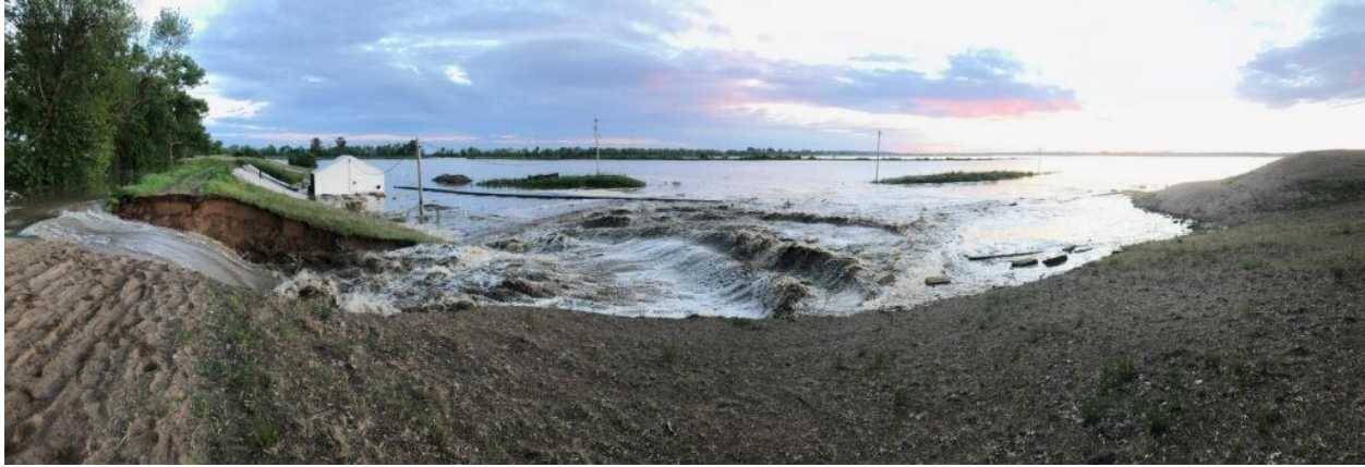
Figure 3.1 Levee overtopping leading to breach (Source: USACE Rock Island District 2019 Mississippi River Flood Fight digital photo library)
